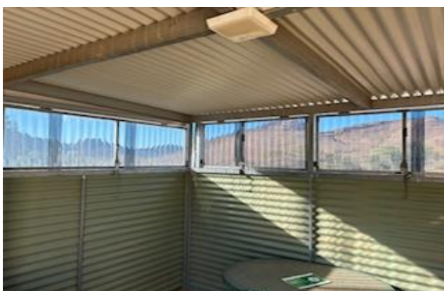
Photo 6- the recently installed shutters on the camp kitchen
